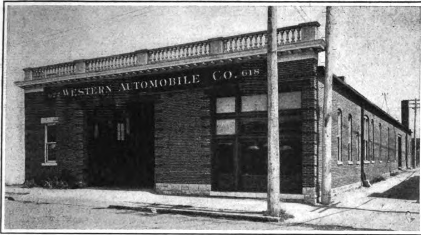
FRONT AND SIDE VIEW OF THE WESTERN AUTOMOBILE CO.'S GARAGE.
